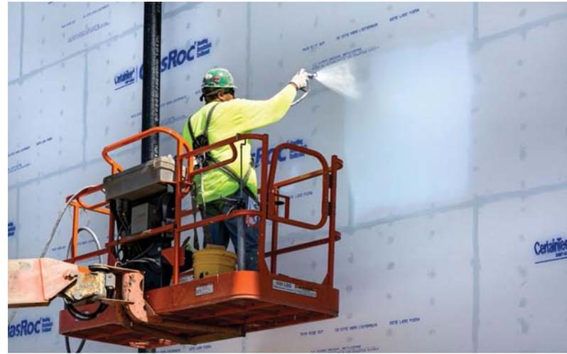
*Dow Corning*® DefendAir 200 was applied to the building’s *GlasRoc*® Sheathing and concrete block substrates using an airless sprayer. Thanks to the product’s excellent unprimed adhesion to most common construction materials, no primer was required.
